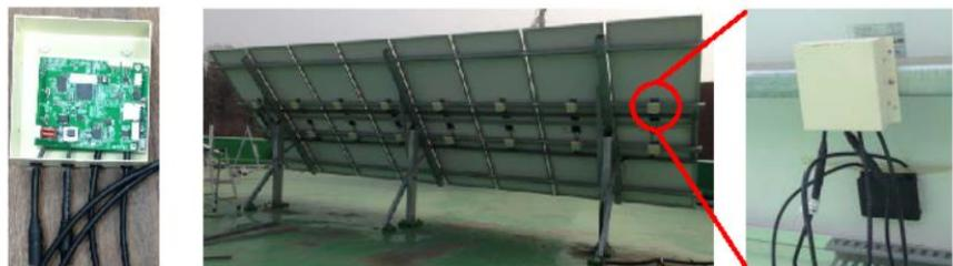
9. Field installation. PLC modem without cover (left), PV modules on
