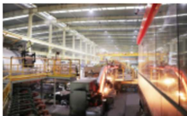
美国连铸连轧生产线 American Southwire Continuous Casting and Rolling Production Line
